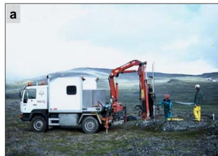
Figure 3. (a) Drilling of Guolasjavri 1 borehole, September 2004. (b) Temperature profile from Guolasjavri 1 borehole, recorded 12.09.2005 (Isaksen et al. in prep). Maximum thaw depth is near 7 m.
